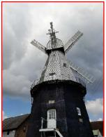
Union Mill built in 1814 was our next visit. It is England's tallest working smock mill. Its white weatherboarded smock tower stands on a tall brick base of three storeys. Four 'patent' sweeps drive one of the two remaining pairs of millstones.
